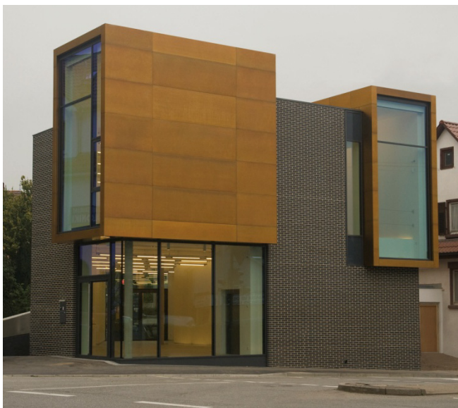
The new building of the ABTART Gallery. Foto: Mark Hindley General plan of the new building: NIXDORF CONSULT Architekten+Ingenieure
